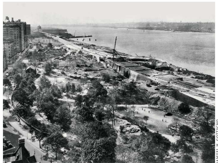
Figure 6 Riverside Park at 82nd Street under construction, showing steel frames installed over the New York Central Railroad tracks, 1936. Milstein Division of United States History, Local History & Genealogy, The New York Public Library, Astor, Lenox and Tilden Foundations
